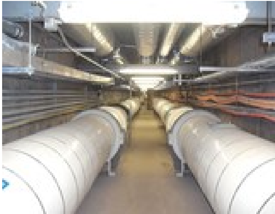
Figure 18.19: Water lines in utility corridors
