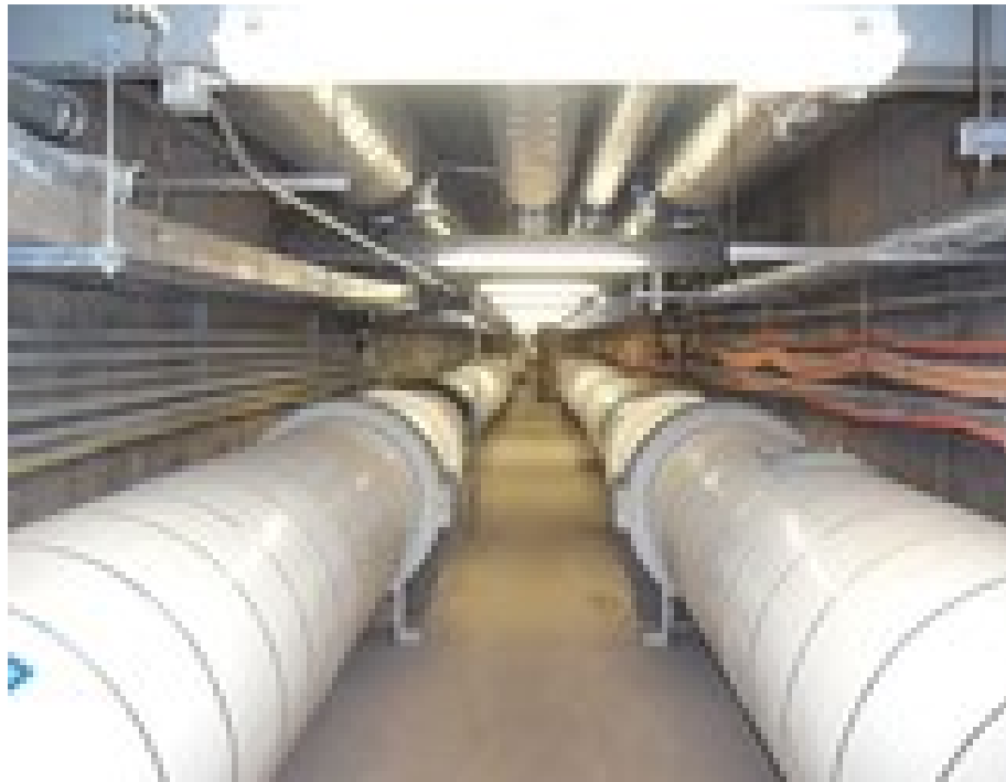
Figure 18.17: Power lines in Utility corridor
