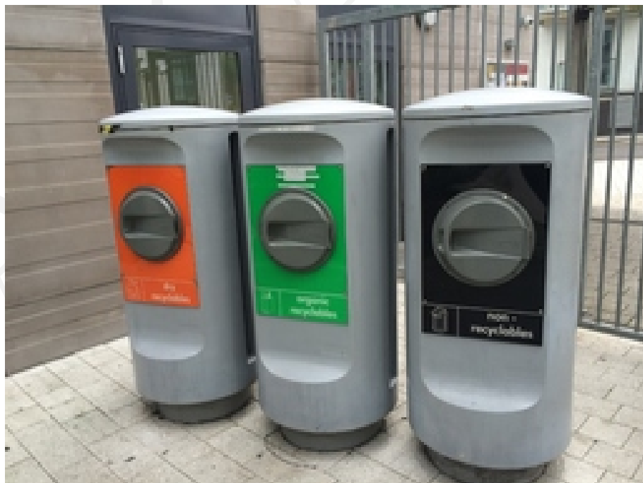
Figure 18.22: Automatic waste collection system with bins
