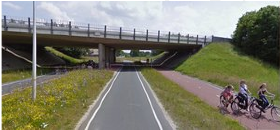
Figure 18.15: Road under bridge (RUB)
