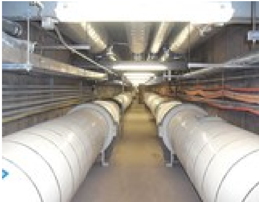
Figure 18.21: Sewer lines in utility corridors
