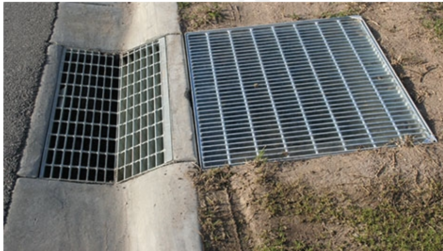
Figure 18.5: Storm Water drainage
