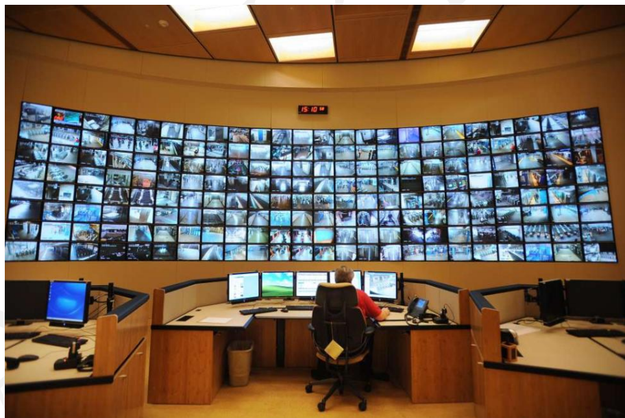
Figure 18.29: Central Command and control center
