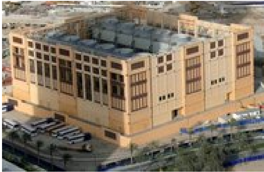
Figure 18.25: District Cooling Plant
